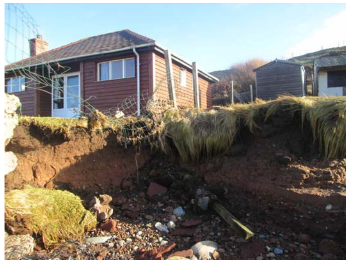
Damage behind defence at Seamill. The most interesting work was undertaken at St Bees promenade, where a sink hole appeared. However, this appeared to have been caused by the stream and not the sea .
